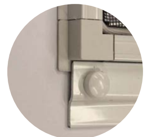
Top and bottom bracket for lift-out screen
